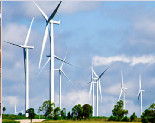
Thai wind project
